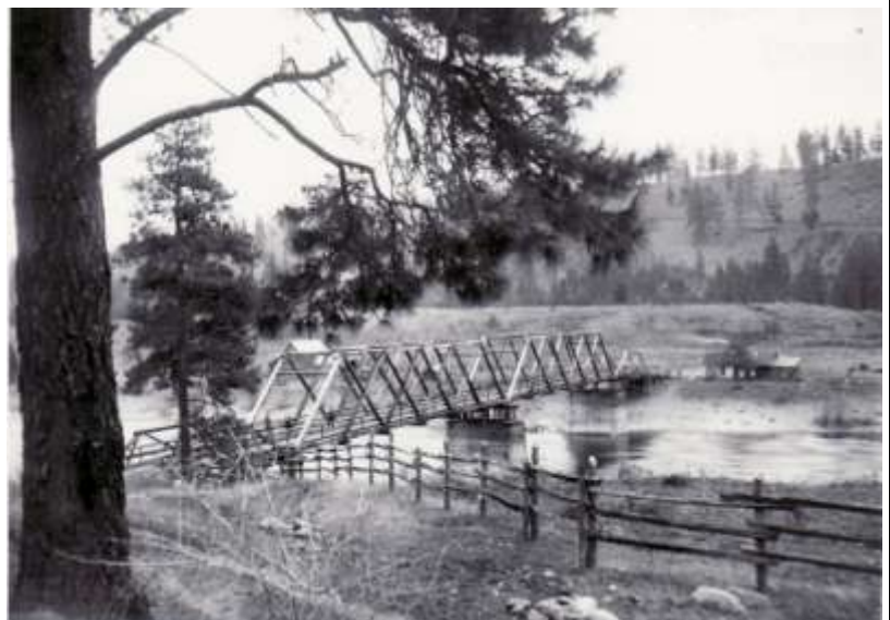
LaPray Bridge, c. 1895
